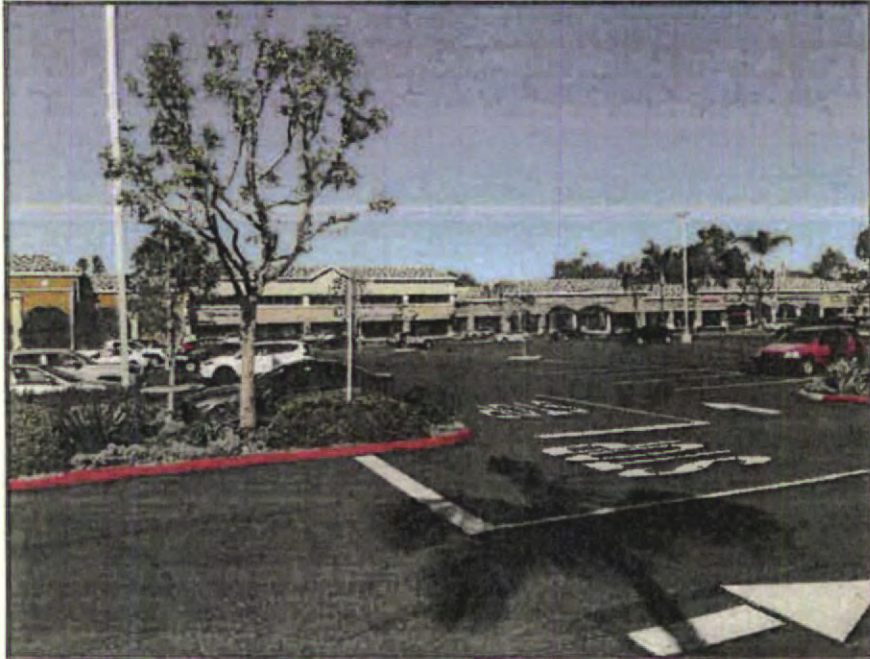
View to the north toward the westernmost segment of the subject parcel.
