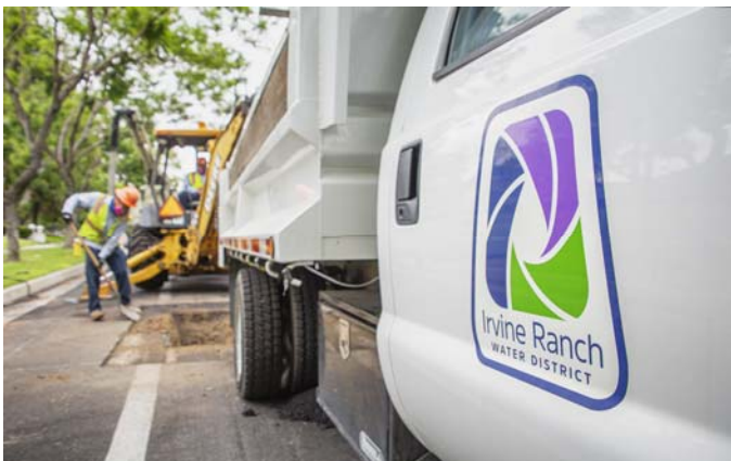
Field Crew on Site
