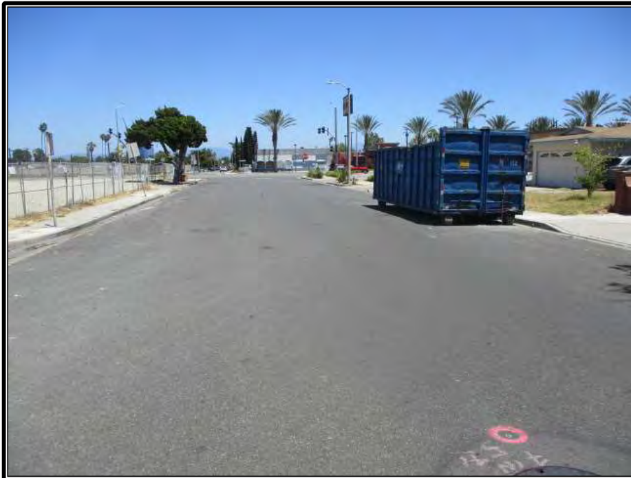
PHOTO NO. 3: View looking east along Twintree Avenue.
