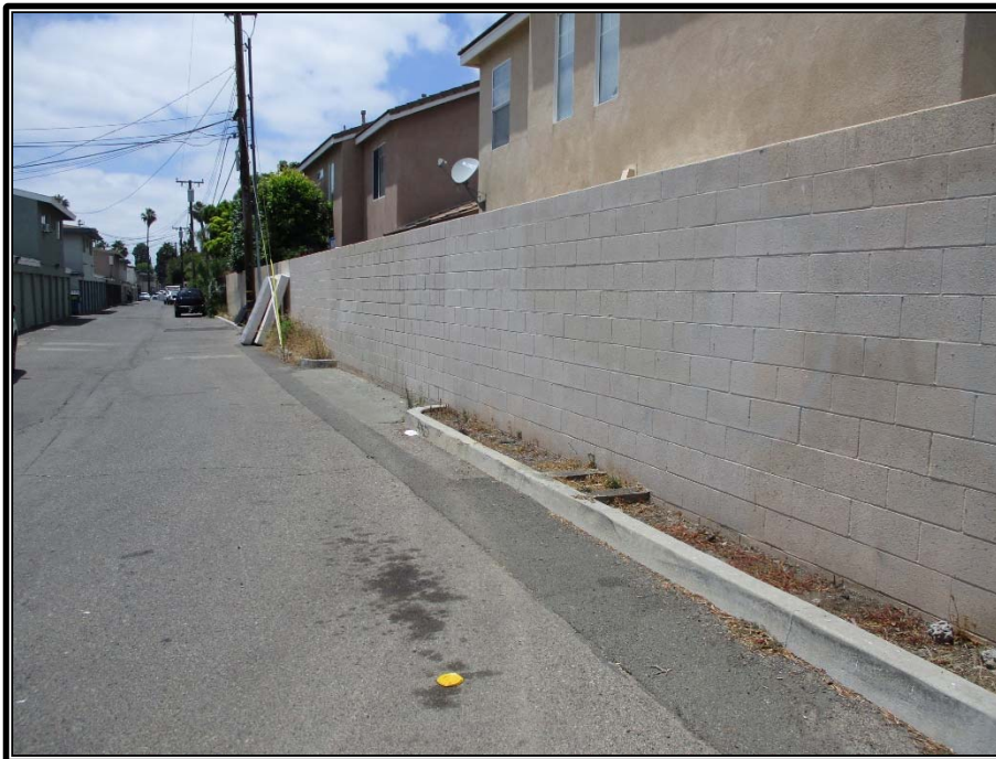
PHOTO NO. 1: View looking westerly at the subject property (portion of alley) from east portion thereof.
