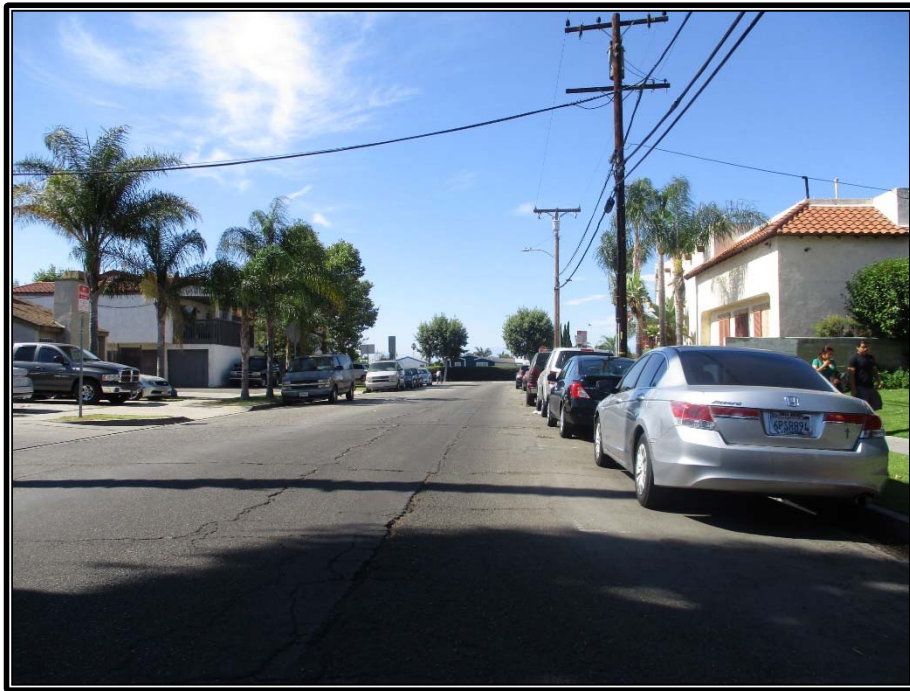
PHOTO NO. 3: View looking south along Rockinghorse Road from a point adjacent to the public alley.
