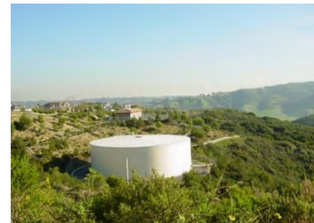
Aliso Viejo Recycled Water Reservoir
