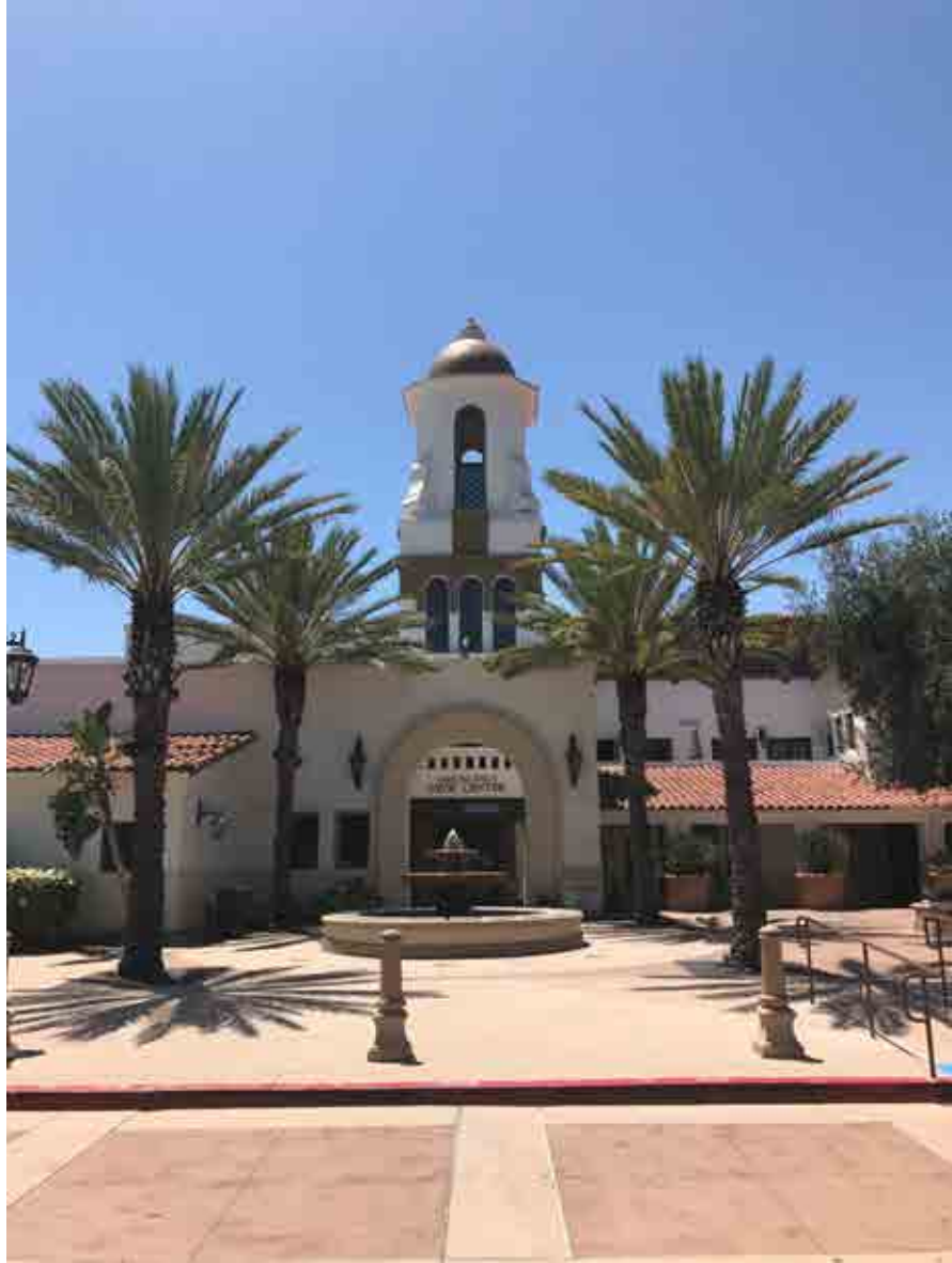
Clerk-Recorder South County Branch Office
