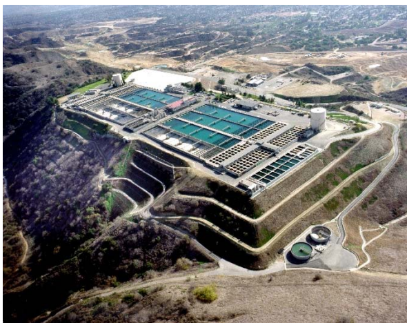
Diemer Filtration Plant
