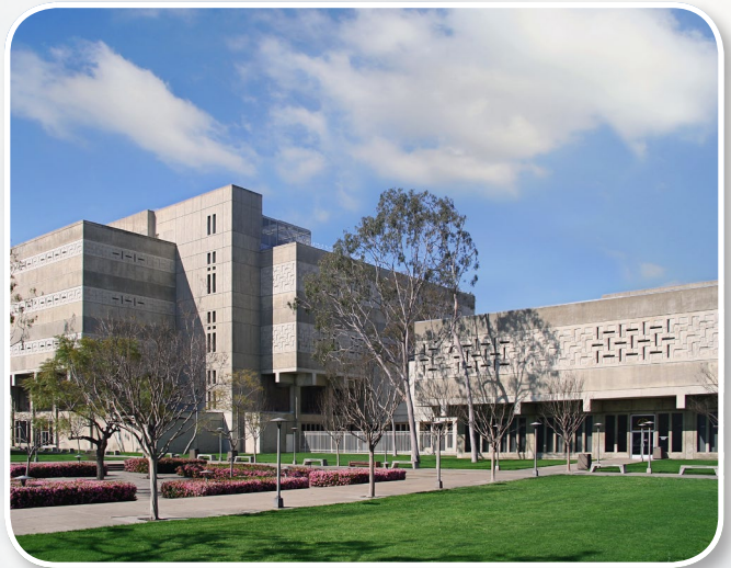
CENTRAL JAIL COMPLEX
